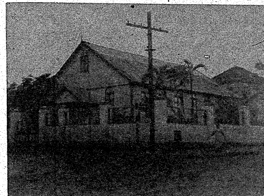
Kingston Church as repaired
