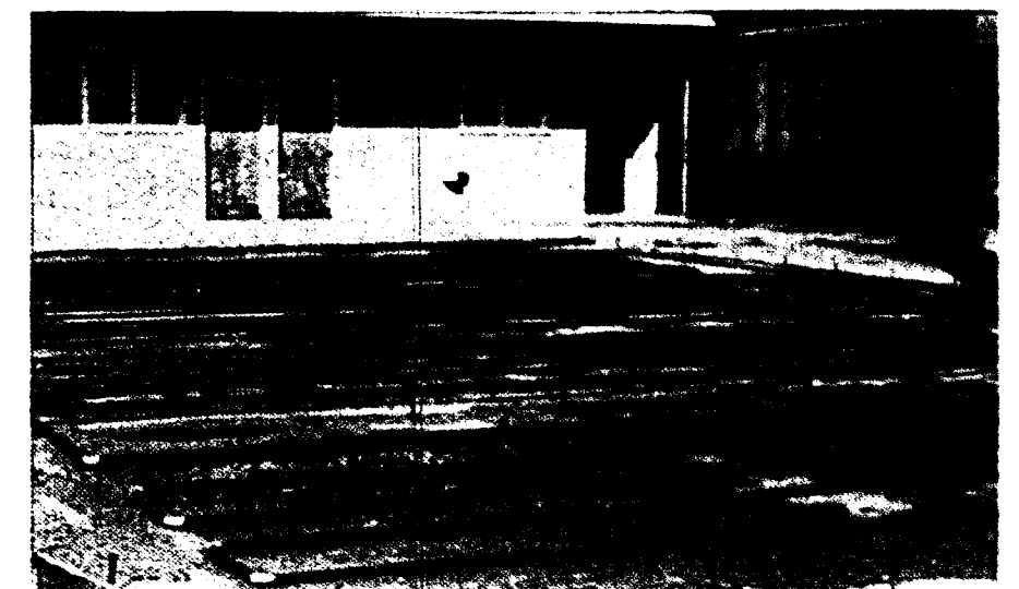
Top: pouring the sub floor of the new building. Bottom: heating pipes ready for covering layer of concrete.
