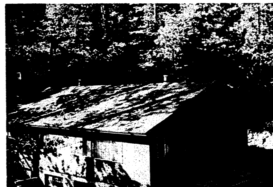
Miller Cottage, a fully equipped, two-apartment dwelling for cooks and staff, recently completed.
