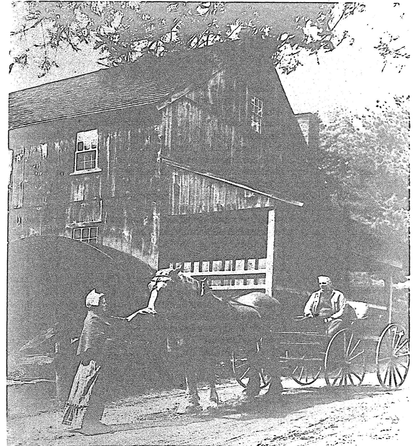
The old grist mill with its undershot water wheel still grinds its corn, wheat, rye, and buckwheat at Sturbridge, Mass., to remind visitors of the earlier days when life was harder but not less happy. Happiness is a matter of faith more than circumstances.
