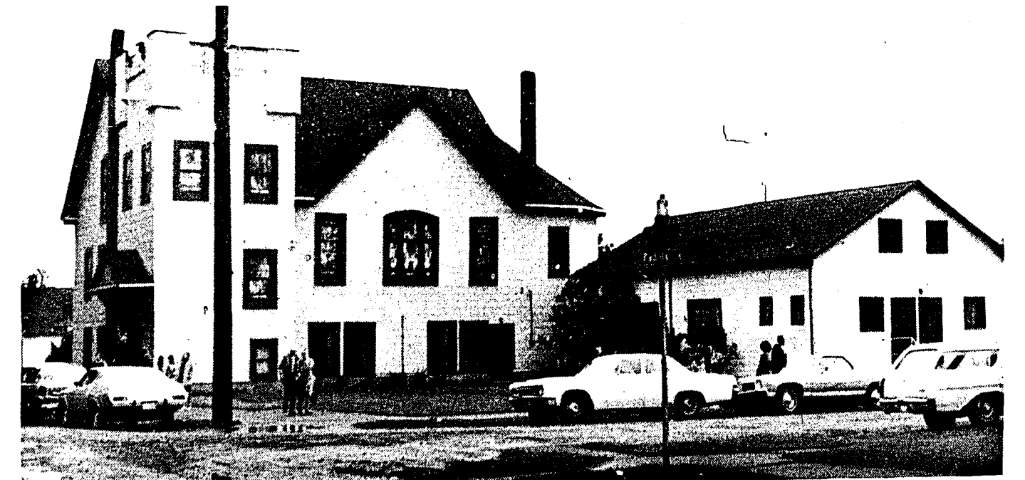
New home for the Seattle Area Seventh Day Baptist Church
