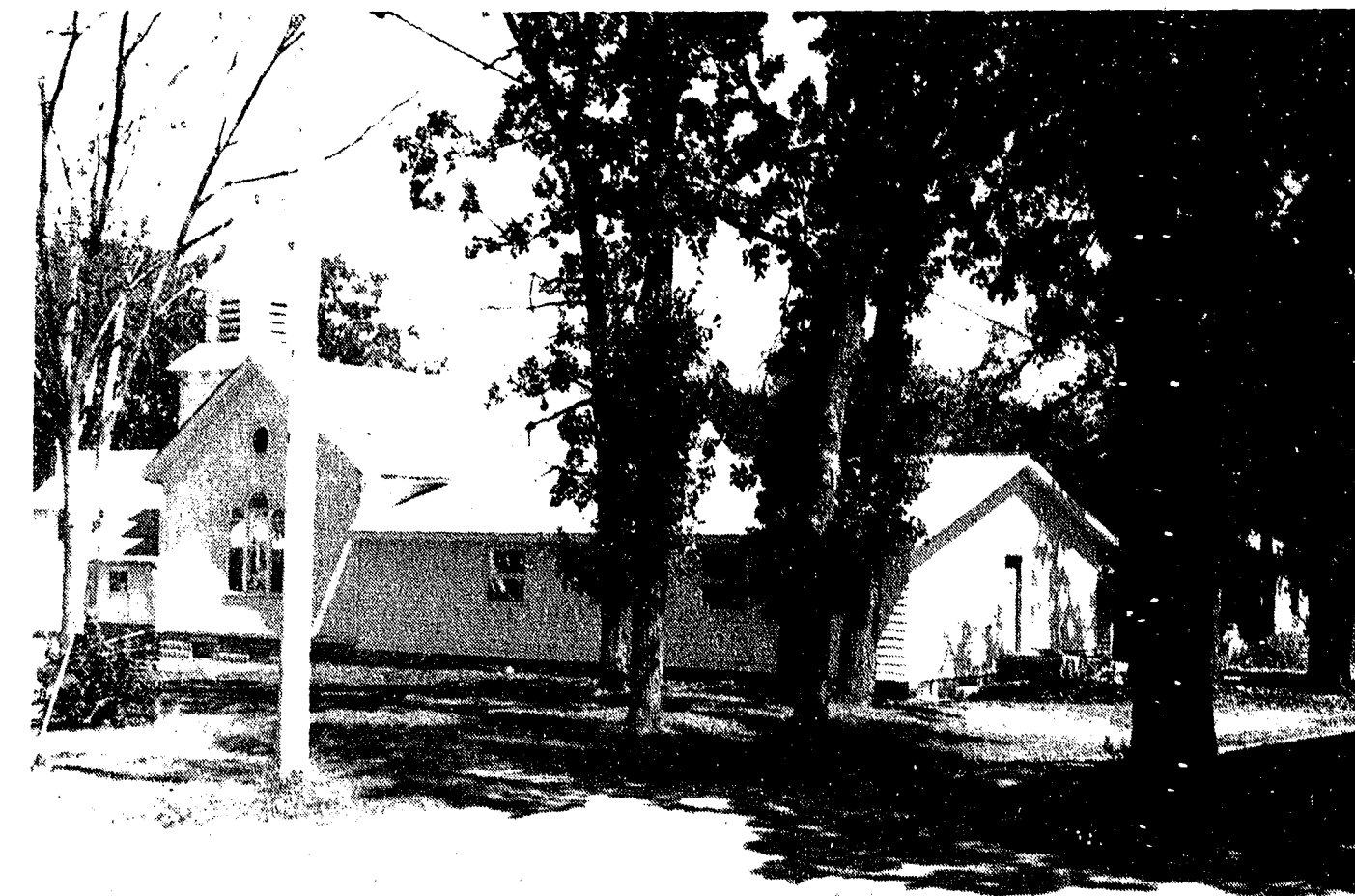
The Dodge Center, MN, SDB Church has completed construction of an addition to the church. The new section provides an assembly room, Sabbath School rooms, rest rooms and church office.
