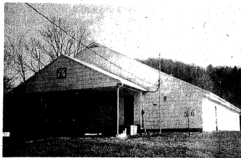
The former Berea school building now houses the main lodge of Camp Joy complete with kitchen, meeting and sleeping accommodations. A new roof and porch are now complete.
