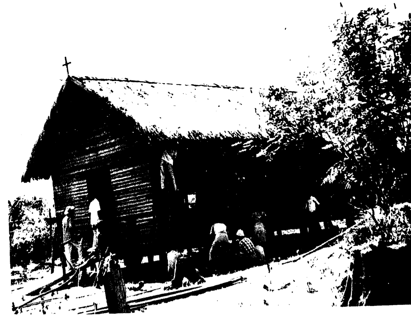
Volunteer workers building the Graca, Burma, SDB Church.
