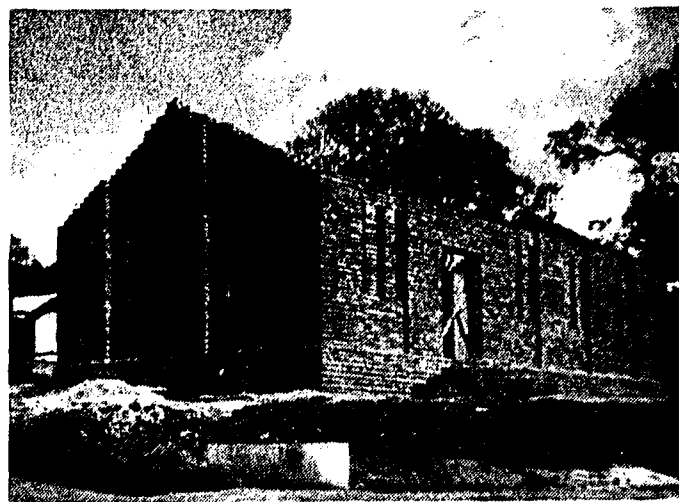
New Mzuzu Church Building: completed to this point by early November 1980, was to have its roof early in 1981. Pastor Harawa is pastor and director of the Northern Association of SDB churches.
