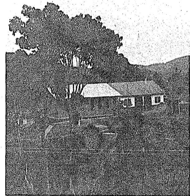
Makapwa Medical Centre with the new Maternity Ward building in the center (light roof).
