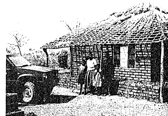
Pastor Matalwera and family next to a new house in the Phalombe disaster area. The structure was built with American funds. To the left is the Makapwa SDB ambulance.
