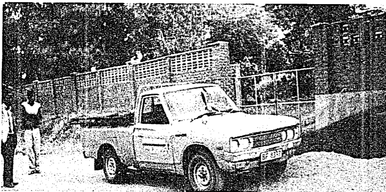
The new brick fence gives security and privacy to the mission house in Malawi.
