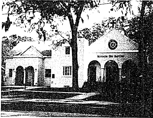
The Daytona Beach church doubled its available space with the new addition (left)—completed just in time for the conference.
