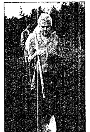
Trustee chairperson Mary Jane Reid steadies the "Golden Shovel" at the groundbreaking.
