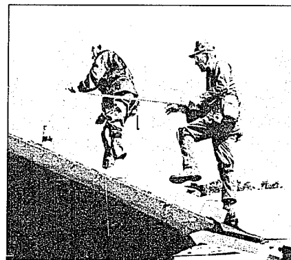
Dale Hull and Phil Watson scale the roof. (Now, turn the photo 90° to the right and think of the old Batman and Robin TV show...)
