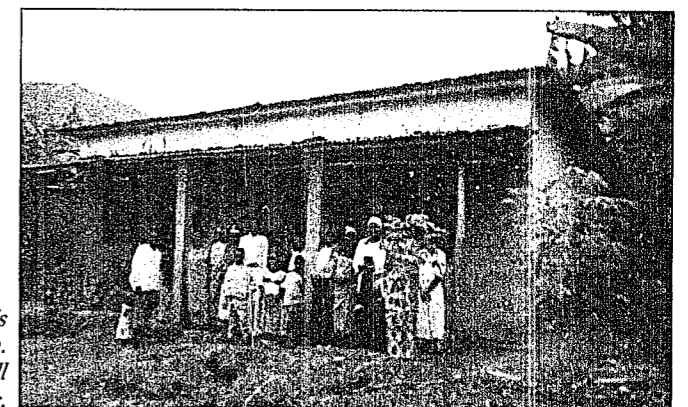
The new Kanama SDB Church still needs doors and windows, but its members are happy to have a proper shelter. Metal sheets currently protect the furniture inside the building.
