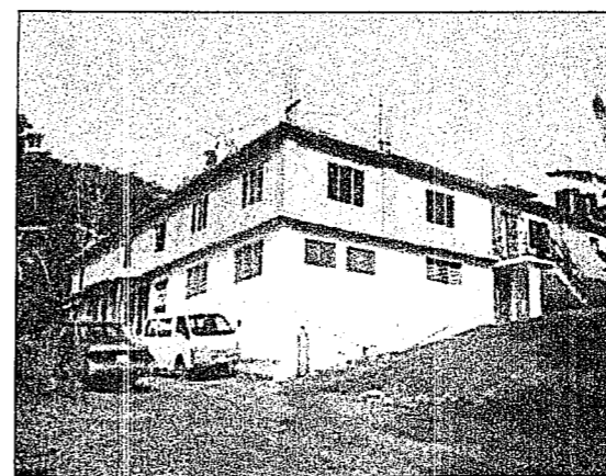
Most of the work was completed on the Maiden Hall Conference Center before the celebration.
