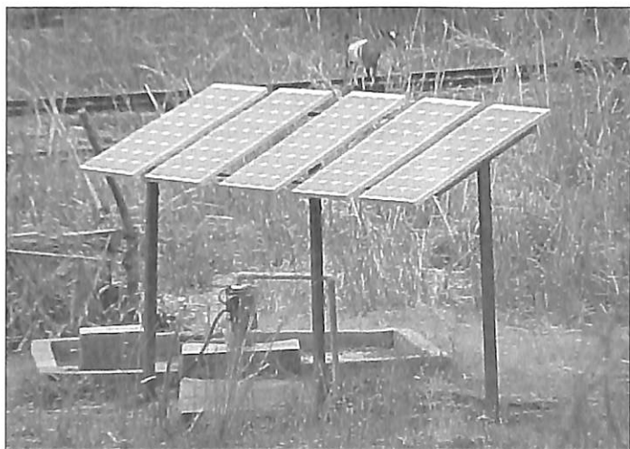
Many solar panels like these were damaged by a windstorm. They run the pump for the water source.
