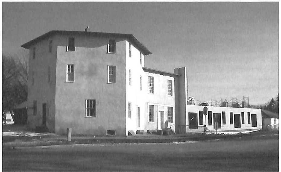
The Milton House is undergoing both renovation and expansion.
