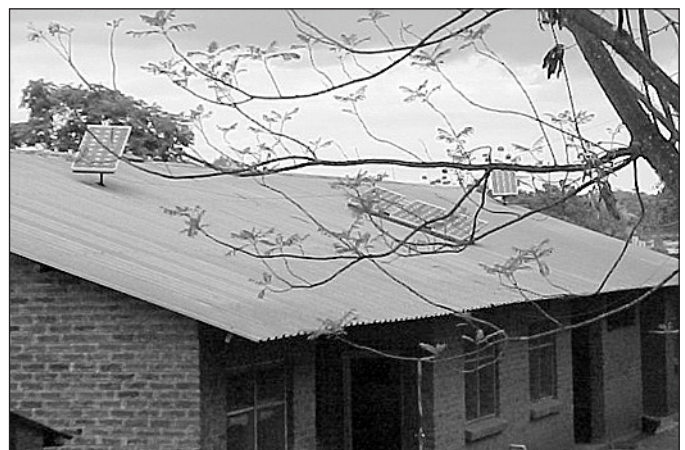
Solar panels are placed on most of the buildings at the Chipho Clinic in Malawi.
