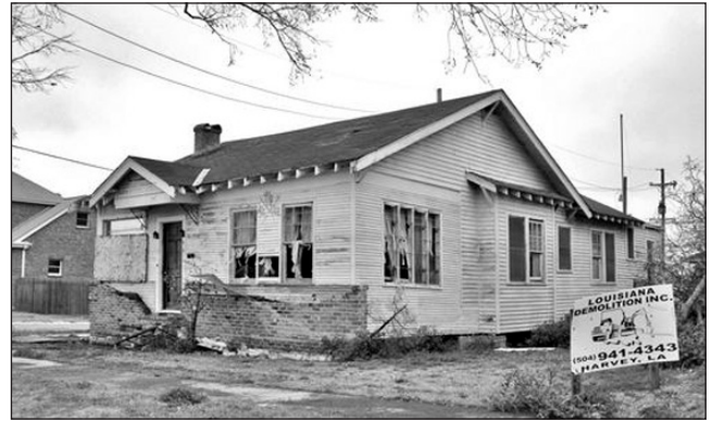
Thousands of houses were marked for demolition.
