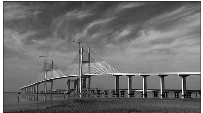
The Sidney Lanier Bridge under construction.
