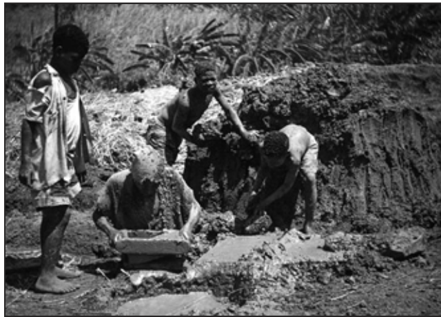
Workers dig up the clay and dirt. Then water is added and the mud is placed in a mold.
