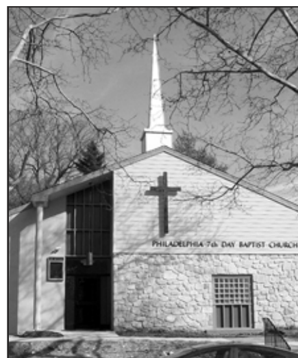
Founded nearly 25 years ago, the Philadelphia SDB Church has undergone major renovations.
