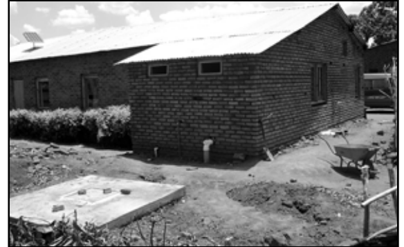
The new Thembe maternity ward extension.
