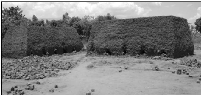
Two of six new kilns making bricks for Malawi SDBs.
