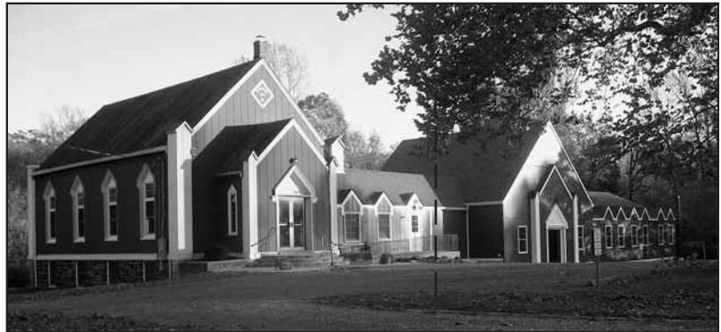
A “quick” construction job, 50 years in the making. The Marlboro SDB Church is enjoying their new addition (right of the dashed line).
