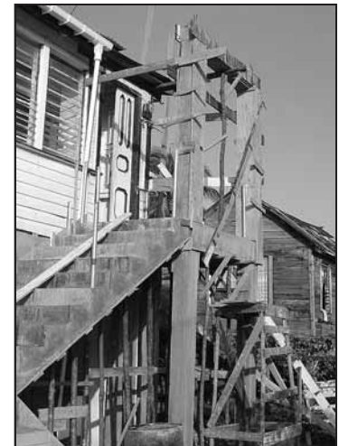
Waiting for the new concrete steps to cure.
