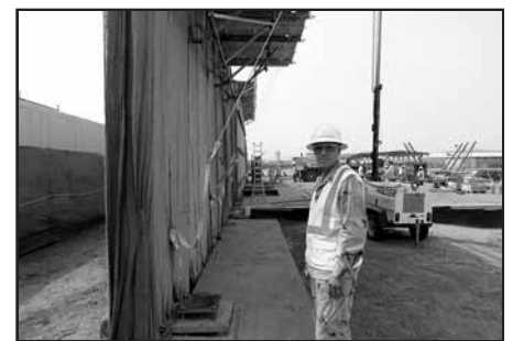
Working at a construction site.
