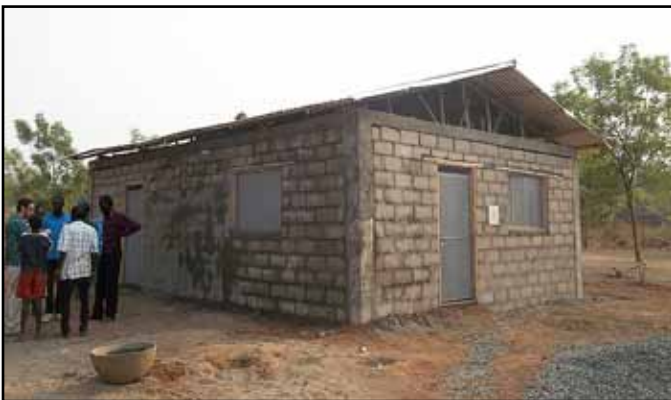
This church building in Gambela, Ethiopia was constructed during the three-week mission.
