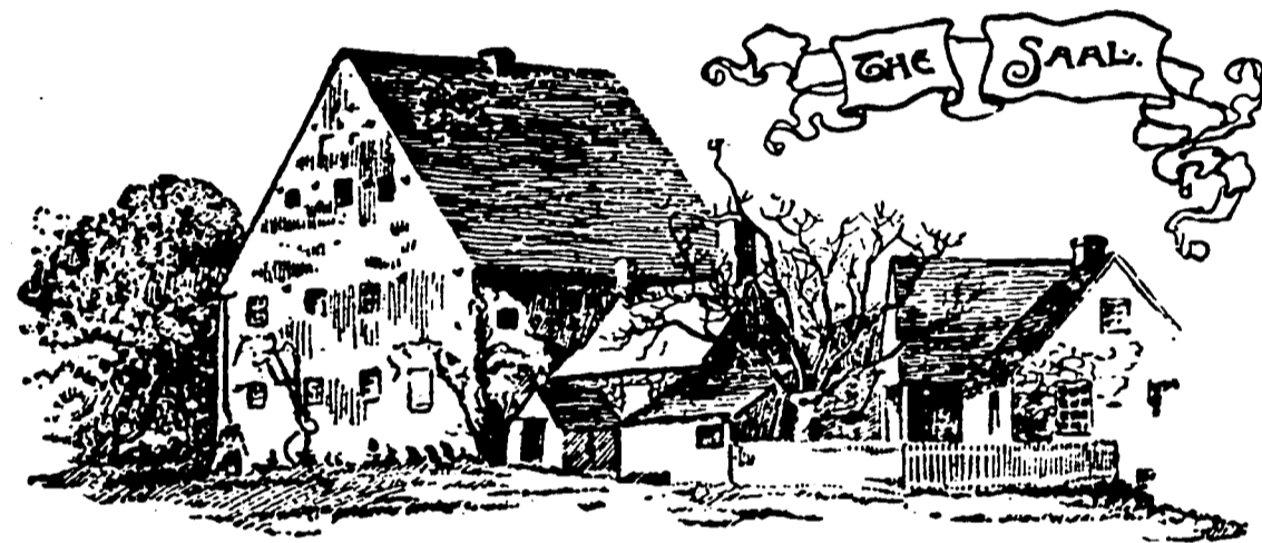
THE SAAL AND OUTBUILDINGS.
