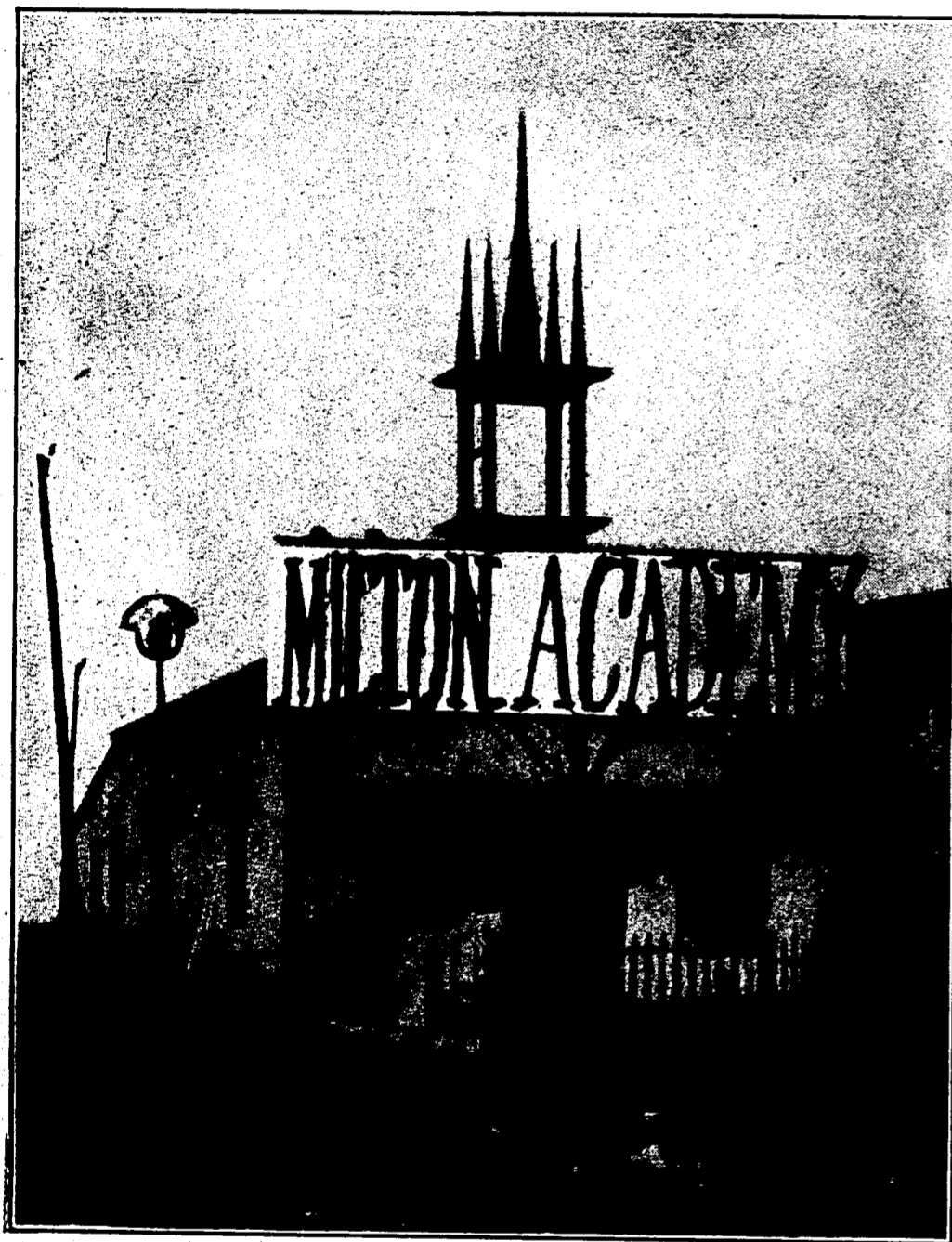
Built in 1844 by Joseph Goodrich, the Founder of the Village of Milton. Used for school purposes from 1844-1855.
