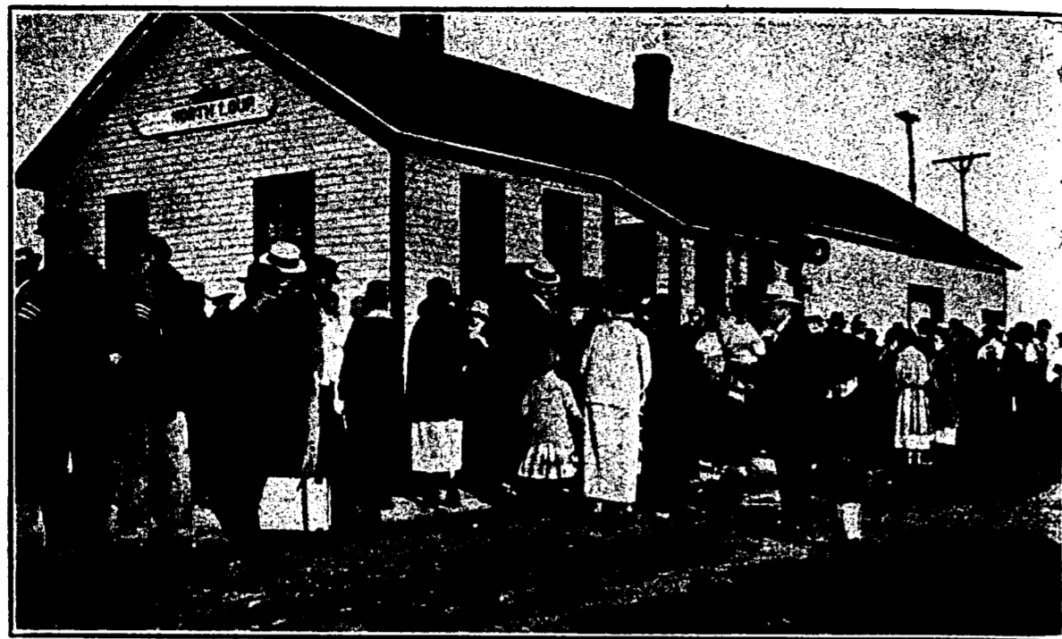
No. 6. Waiting for the Train—Morning After Conference
